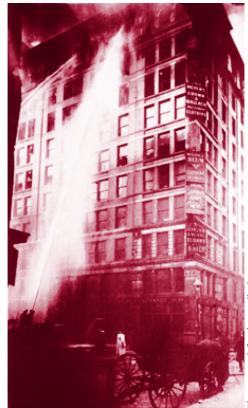
Fire fighters struggled to extinguish the burning Triangle Shirtwaist Factory. Fire-quenching sprinkler systems, though proven effective, were considered too costly by many factory owners and were not installed in the building.
