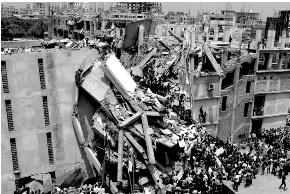
The Rana Plaza building in Bangladesh
